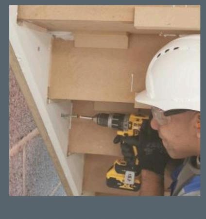
These fixing points highlight where stairs should be fixed and allow simple on-site quality checks during the build process to diminish the risk of squeaking stairs and potential customer care issues post occupancy.
