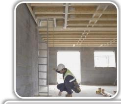
Measure the actual finished floor height and check this matches the Label.
