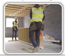
2 Load the staircase into the plot and ensure it is stored on bearers (wall string down). Check for any signs of damage.
