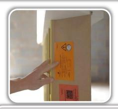
3 Check the stair is in the correct plot and note the finished floor height shown on the Traceability Label.
