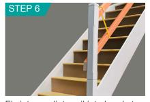
Fix intermediate rail into brackets using 4 x 40mm screws. Important – please ensure the minimum 80mm overlap of the newel is positioned on the side shown above.
