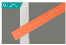
Cut intermediate rail to length leaving a minimum of 80mm overlap of the newel at both ends.
