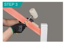
Using batten strike down until rail is fully locked in position.
