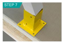
Fix balcony post into universal post bracket and fix at each end of opening.
