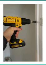
**Note:** If a dummy Door is supplied, fit by removing the screws and adjusters from the female hinges, then slide the Door into place over the male hinges and re-fit the adjusters. Make sure to check the frame is still square and adjust as needed.
