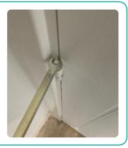
**Note:** Doorstops are reversible and can be positioned according to the thickness of the Door (35mm or 44mm). All stops should be pinned and glued in place using 38mm long pins. Before installing Doorstops ensure the frame has been permanently fitted to the supporting walls using 75mm long screws at maximum 600mm centres.
