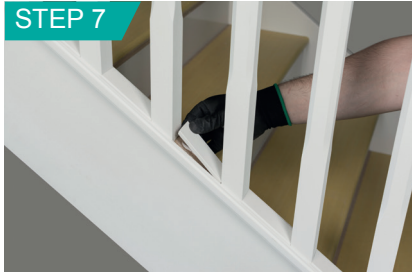
Fit infill with PVA glue.
