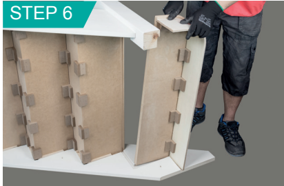
Fit bullnose tread into position.
