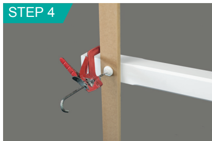
Support end of newel-post to ensure it remains square during assembly.
