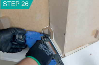
Position blocks and secure with mechanical fixings.
