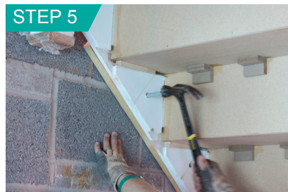
Fix stairs to wall using fixings specified by the housebuilder (not supplied).
