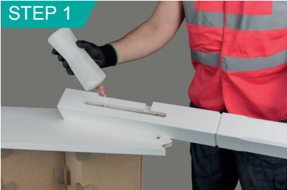
Glue machined mortise in bottom newel-post with PVA.
