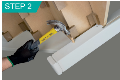
Knock dowels into pre-drilled holes.
