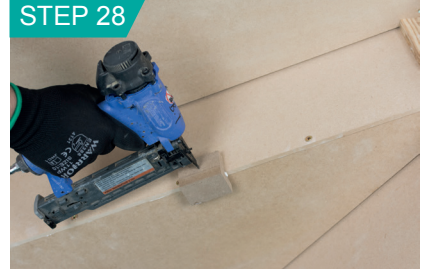
Position block and secure with mechanical fixings.
