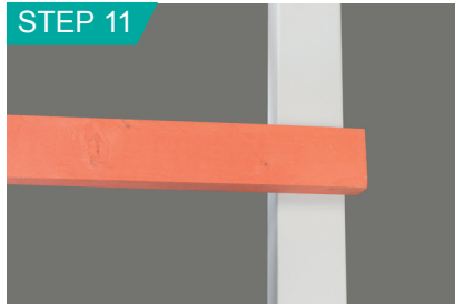
Cut intermediate rail to length leaving a minimum of 80mm overlap of the newel at both ends.
