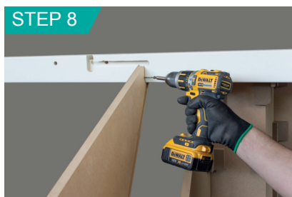
Fix firmly in place by screwing to newel-post.
