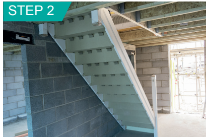
Position stair ensuring the treads are level.
