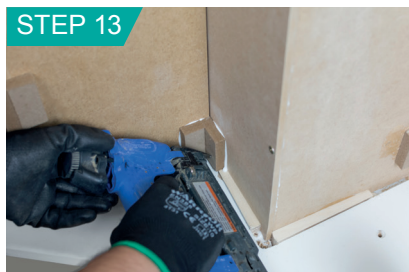
Apply PVA glue to inner corner where tread and riser meet and attach glue block.
