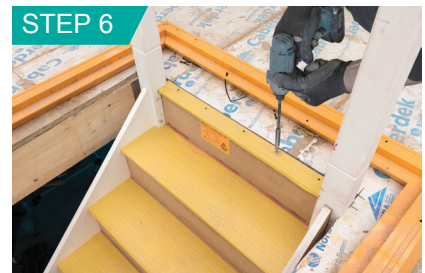
Fix nosing to trimmer.
