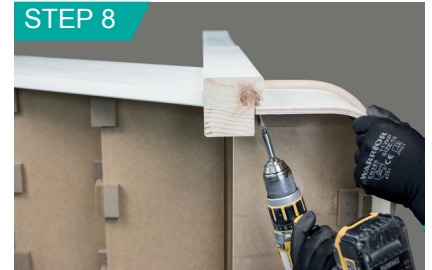
Screw riser and tread into newel-post.
