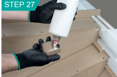
For glue blocks on outside angle, apply glue to inside of block.
