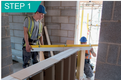
Ensure newel posts are fixed square to the tread.
