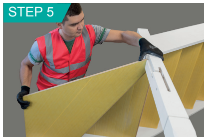
Slide treads into pre-routed housing on string.
