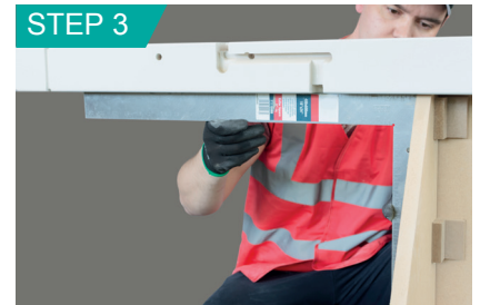
Check for square in both directions against tread.
