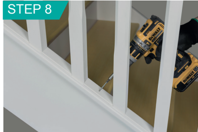
Fix through infill using a screw and cup and leave exposed.
