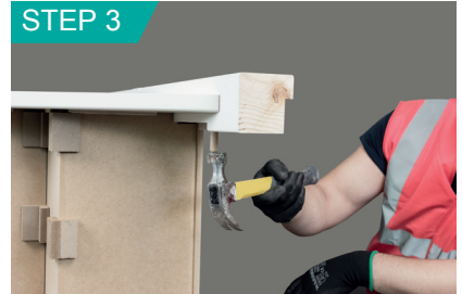
Knock dowels into pre-drilled holes.
