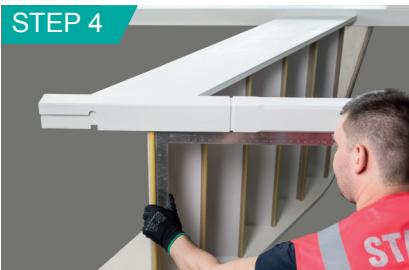
Check for square in both directions.
