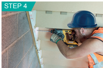
Use pre-drilled holes as a guide and drill for fixings.
