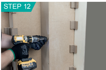
Screw riser to back edge of tread.
